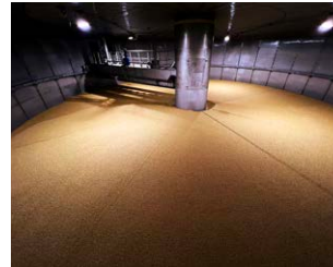
2022 Groundbreaking new kiln.
